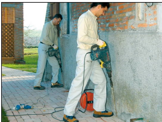
Photo 7. Phase de perforation
