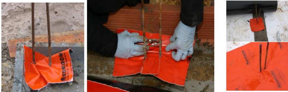
Figure 18 – protection des ferrillages
